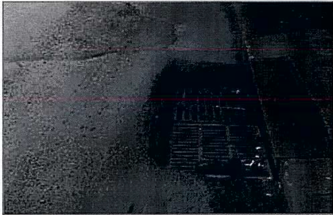
Below-grade drain grates create hazards for bicyclists.
